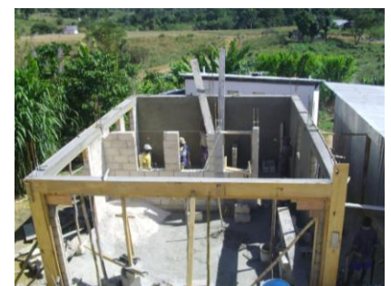
Top: Public well in LaTwazon Bottom: Construction of incinerator
